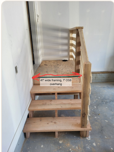
Framed landing, rail set, ready for finish
